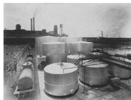
Tank Farm and filling equipment
